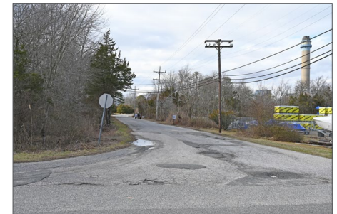
5. View looking northwest from North Shore Road toward the Clay Avenue access road to the proposed BL England Substation site.
