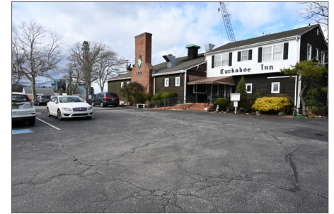
2. View looking north at the Tuckahoe Inn. Portions of BL England Generation Station are visible in the background of the image.
