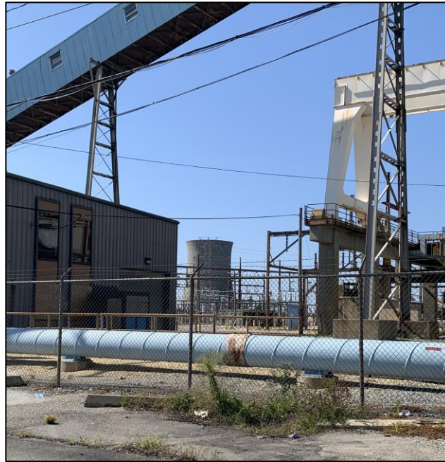
Figure 4 – Cooling Tower, Electrical Substation and improvements
