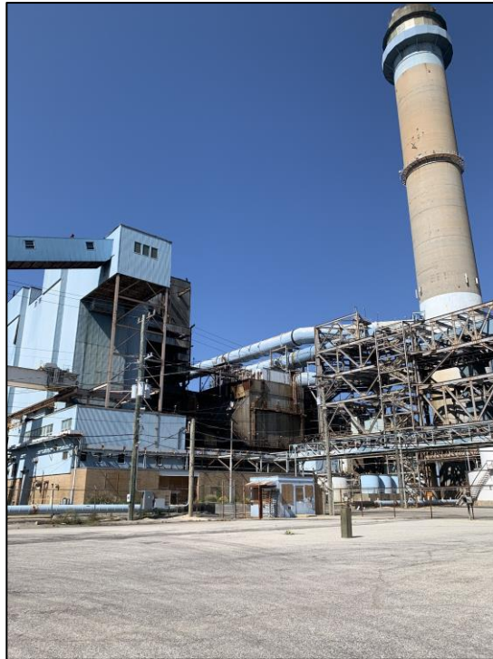
Figure 2 – Air Scrubber, buildings and improvements
