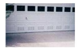
Several manufacturers have developed products that meet the flood venting requirements. Some of these products are certified to enable equalization of water pressure with smaller openings.
