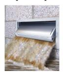
The walls of any enclosed area below the flood protection level must be designed to automatically equalize hydrostatic forces that result from the pressure of floodwaters against the structure. This is accomplished by installing openings, or flood vents, through which water can enter and exit the enclosure to maintain equal levels on both sides of the wall.
