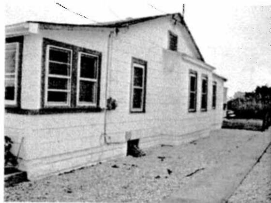
WEST SIDE VIEW 11/26/2013
